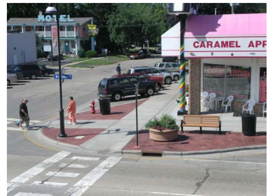
Figure 2. Curb Extension at a Street Intersection
